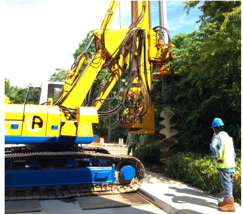
Driving the first pile into the ground
