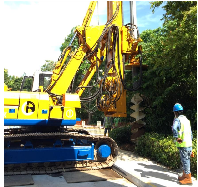
Driving the first pile into the ground
