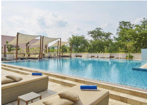
Renovation of swimming pool, pool deck, gym, meeting room
