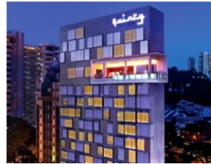
5 The Quincy Hotel (108 rooms)
