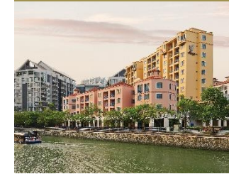
11 Village Residence Robertson Quay (72 units)
