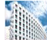
Adina Serviced Apartments Singapore Orchard
