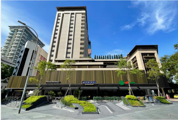
New Ribbon Cladding
