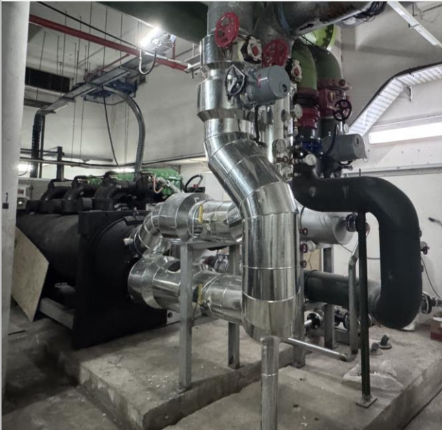
Upgrade of chiller system to improve energy efficiency
